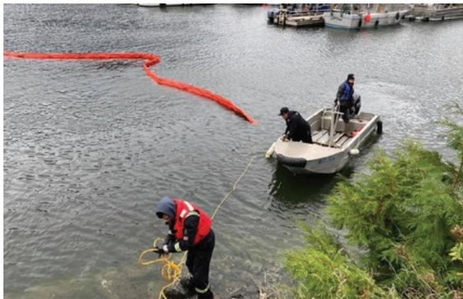
**FIGURE 32:** Guardians deploying oil spill containment equipment (photo credit: Roger Harris).
